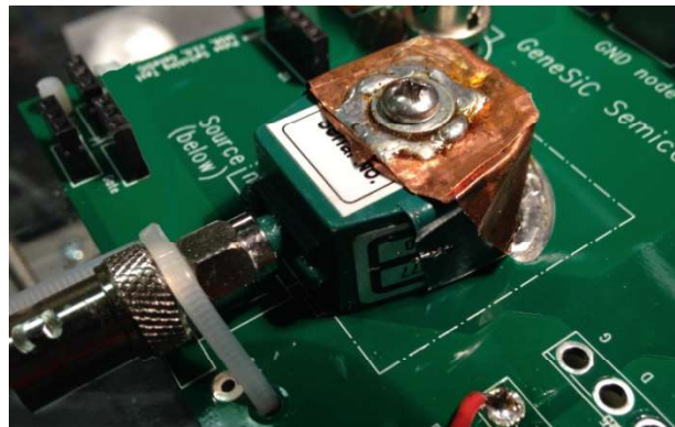
Figure 4: Drain Current Sensor Connection with Pearson Current Monitor installed using a low inductance current path.
