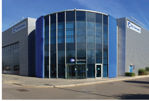
European Headquarters & Production Facility, Southampton, UK
