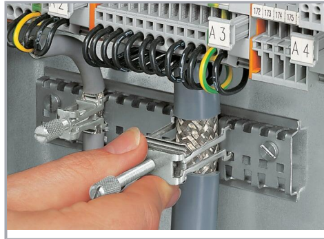
Securing an additional shield clamping saddle.
