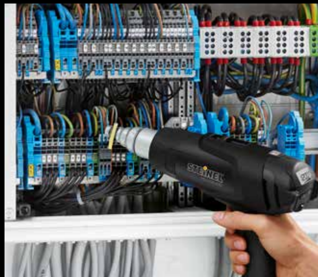
Shrinking cable sleeves in distribution cabinet.
