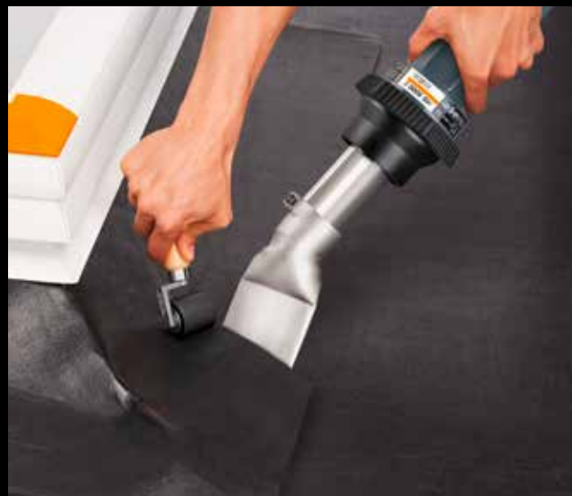
Overlap welding on a light dome.
