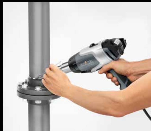
Welding plastic in tank and apparatus construction.
