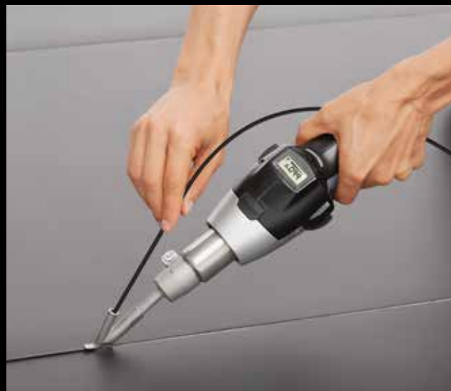
Welding linoleum floors.
