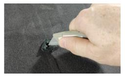
3. Remove the cable grommet with the large opening from the distribution box. Use a utility knife to cut the scored "X" to help pass the cable into the box.
