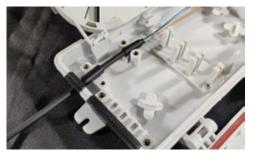
6. Wrap electrical tape around the cable where the cable clamps are located to ensure a secure fit. Make sure the grommet is fit into the body of the distribution box.
